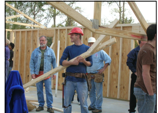
"Sweat Equity" Builds Foundation of Houses and Hope
